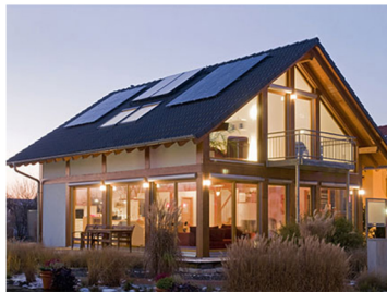
Off grid power system
