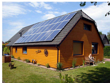
Off grid power system
