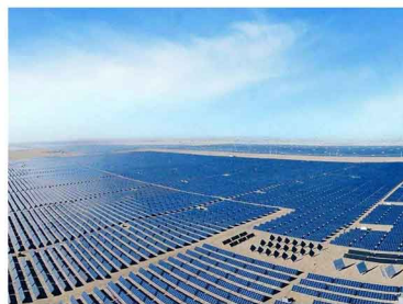
Photovoltaic power station
