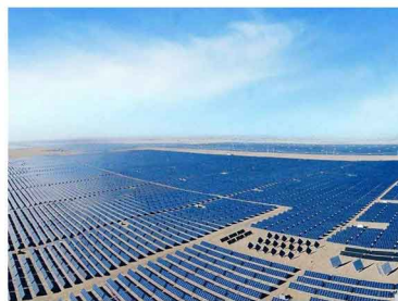
Photovoltaic power station
