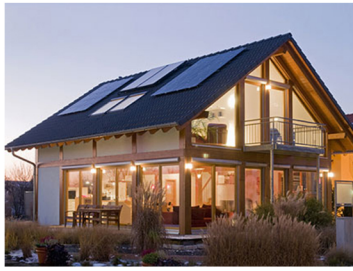
Off grid power system
